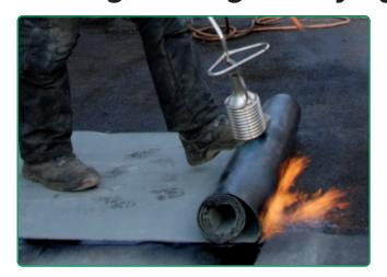
The M2 TURBO is a propane power-roofing torch with brute power and a flame length of up to 95 cm.
